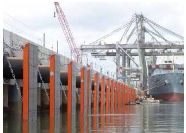
Barbours Cut Container Terminal | Houston, TX | USA
