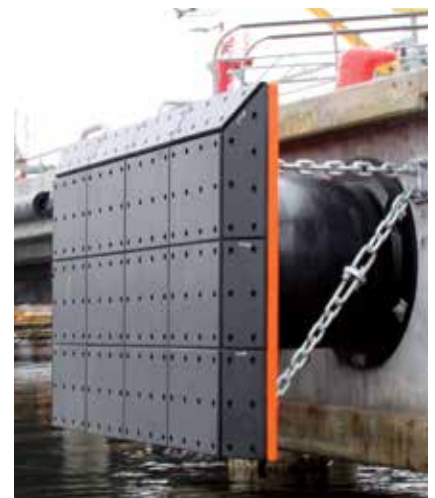
Chemical Product Jetty | Stenungsund | Sweden
