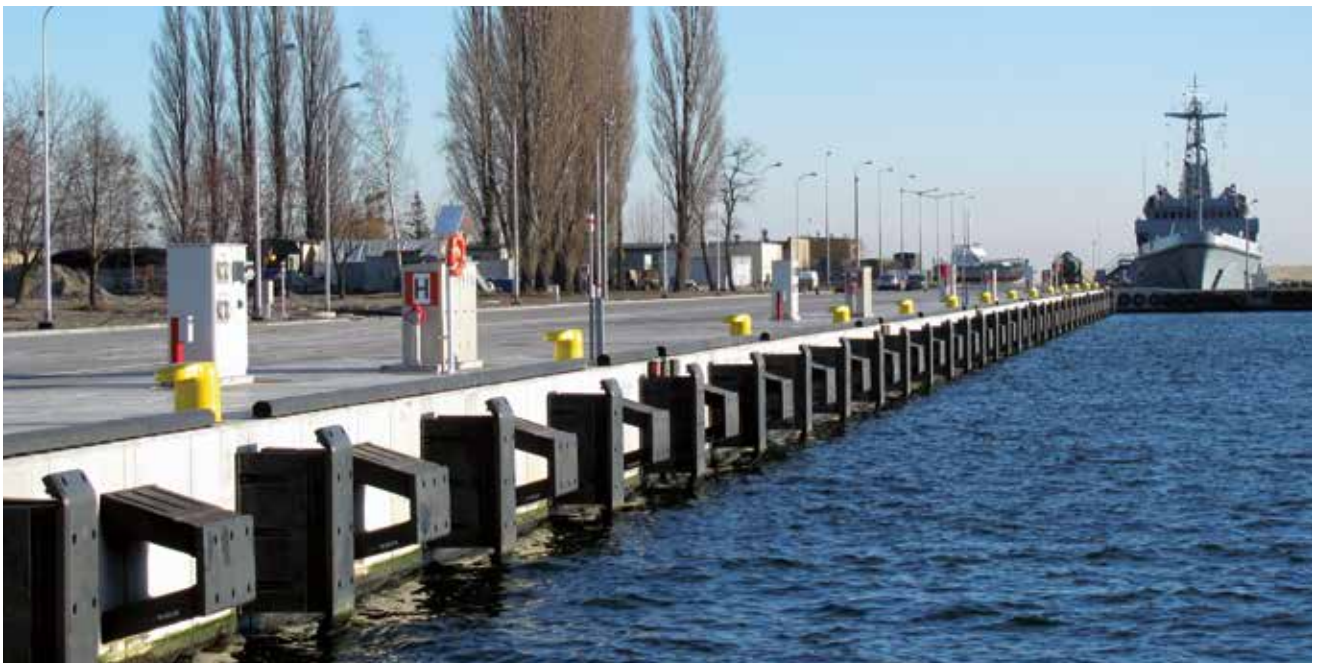
Northern Berth 16 | Port of Gdynia | Poland
