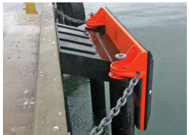
Pier 1 | North Kingstown, RI | USA
