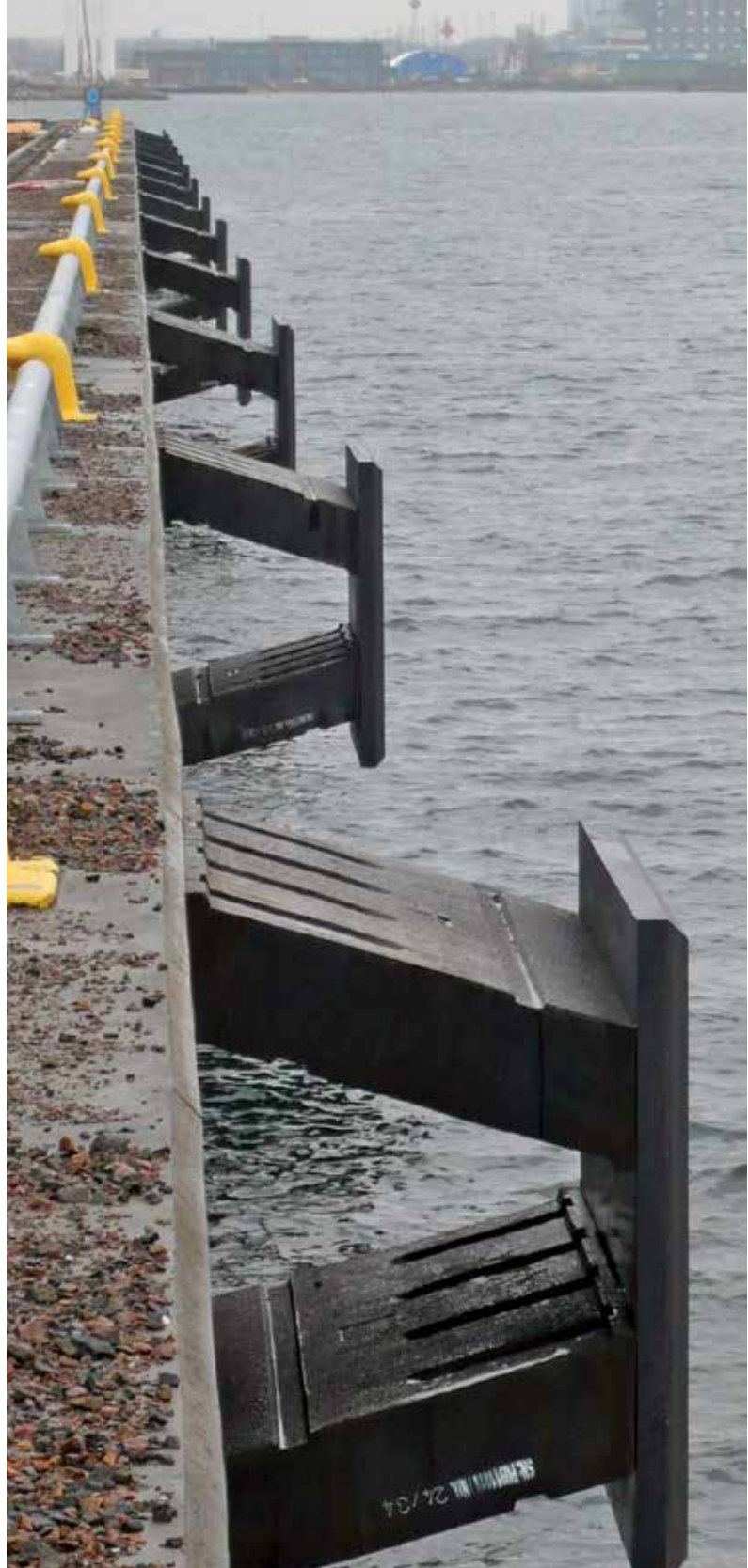
Ferry & RoRo Terminal | Malmö | Sweden
