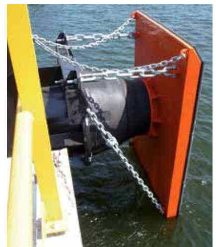
Eurotank Jetty | Amsterdam | The Netherlands
